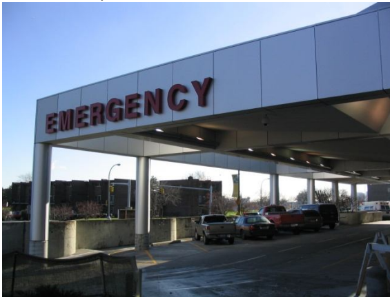
Detroit Hospital, USA, 01
